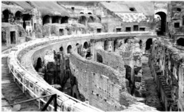
Fig. 1 General view of the podium north wall
