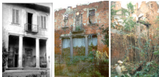
Figure 3: CR: damages evolution of the owner house (1940-'91-'98)
