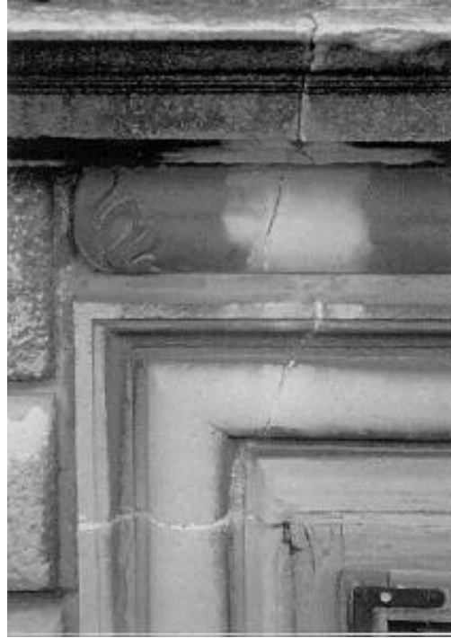
Fig. 2 : A cornice under the balustrade
