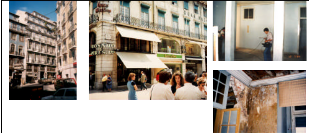
Figure. 1: “Baixa Pombalina” buildings, showing main deficiencies
