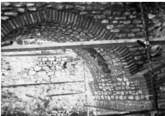
Figure 2: Partial reconstruction of the vaults.
