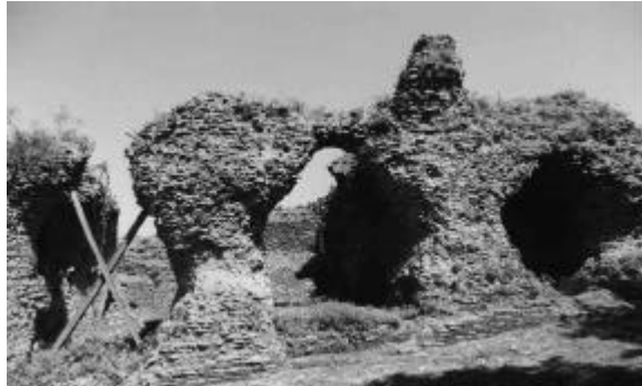
Figure1: The amphitheatre before the restoration.
