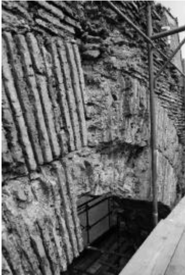
Figure 4: The arch before the reintegration.
