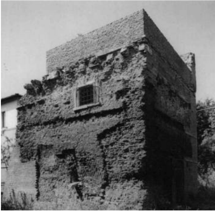
Figure 10: The building after structural restoration.
