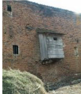
Fig.10: Added eastern toilet [2] Kulla of C. Ahmetaj, Zabllac, Istog
