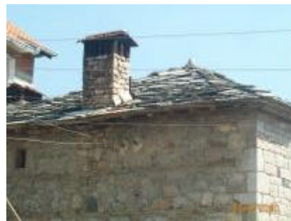
Fig. 6: stone sheet roofing [2]. Kulla of H.Maxharraj Gramnik, Klina
