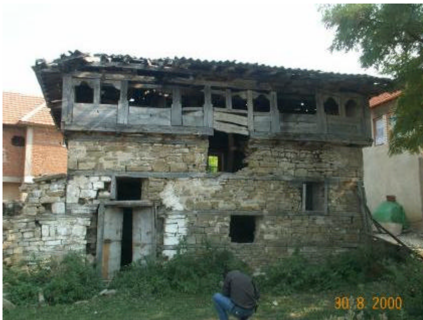
Figure 4: Kulla of S. Mata, Doberdol, Klina, with cardak style cantilever [2].
