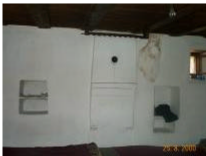
Fig. 7: closed fireplace with hanger [2] Kulla of H. Maxharraj, Gramnik, Klina
