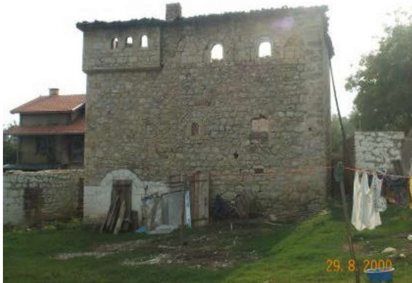
Figure 2 : Kulla of K. Fazlia, Lubozhda, Istog, constructed of stone [2].
