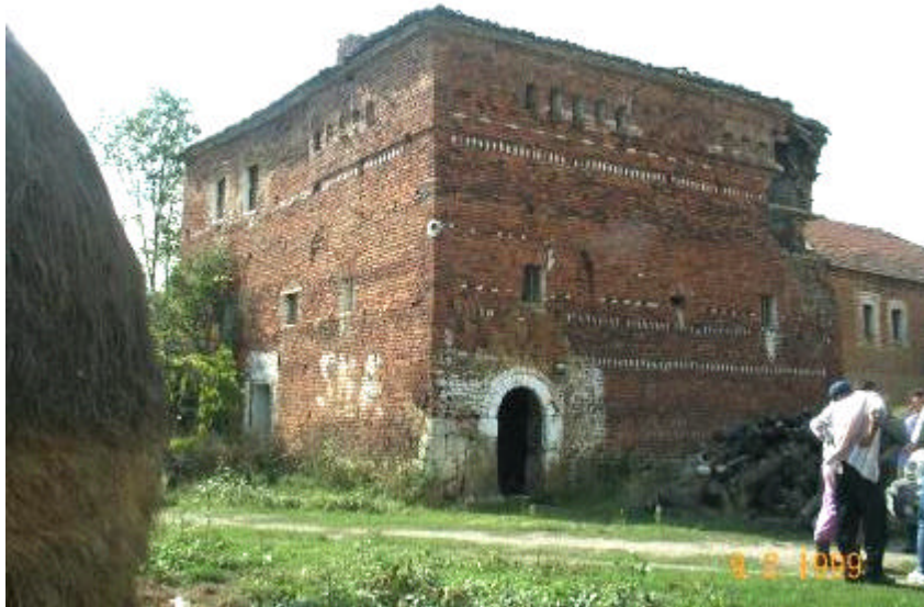
Figure 3 : Kulla of C. Ahmetaj, Zabllac, Istog, constructed of brick [2].
