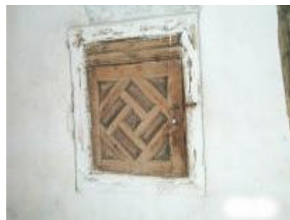
Fig. 8: built-in cupboard [2] Kulla of U.Ukaj, Kaliqan, Istog
