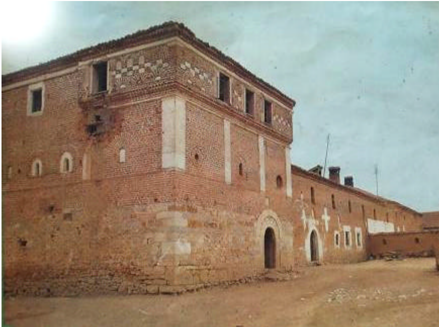
Figure 1: kulla of M. Gega, Gjurrakoc, Istog, as it used to be with the attached annex. Constructed of stone and brick. Taken from an old picture [2].
