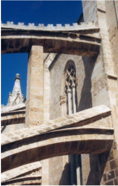
Fig. 3 – Flying arch propped on a masonry column
