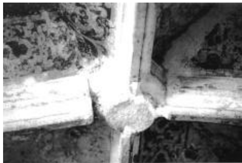
Fig. 5: Intradosal crack in the rib section
