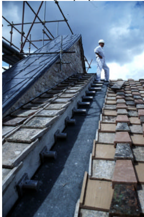
Fig. 4 : The three sets of installed SMADs
