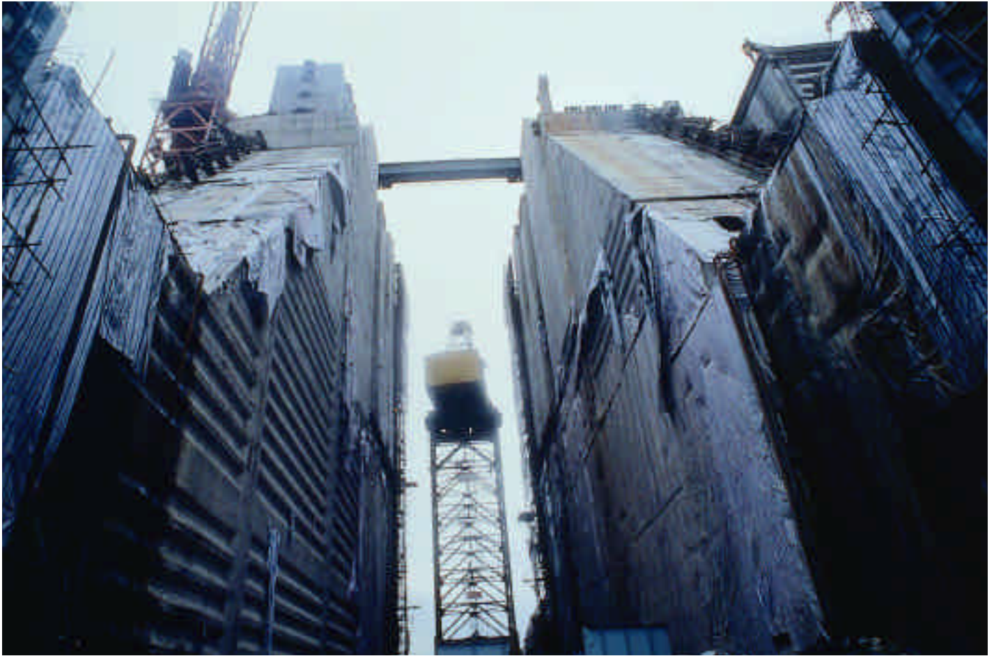
On the rise: construction of a dam as part of the giant Three Gorges project on China's Yangtze River.
