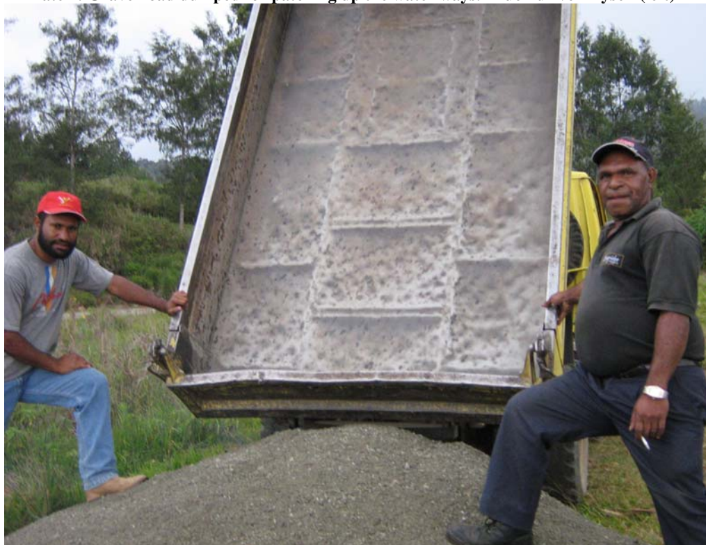
Plate 7: Gravel load dumped for patching up the water ways. Truck driver myself (left)
