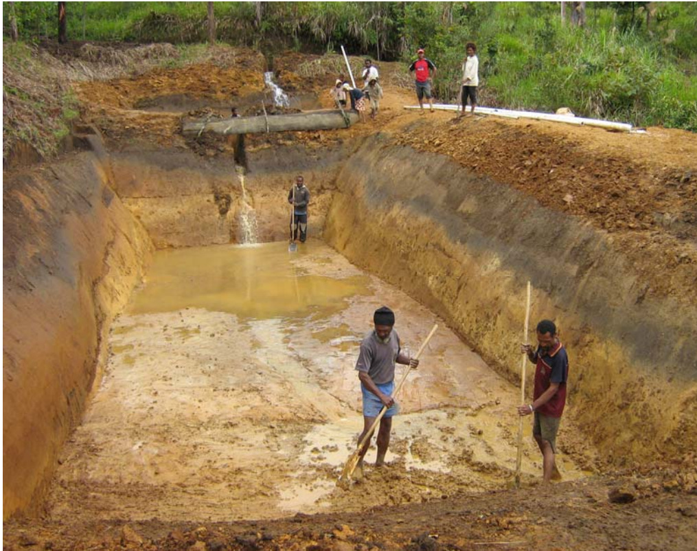
Plate 3: Engaged carpenters doing the final touches before the water fills the ponds
