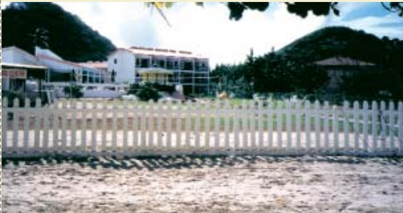
This hotel at Grand Anse, was positioned well behind the dynamic beach area and was safe from Hurricane Lenny's waves, Nov. 1999
