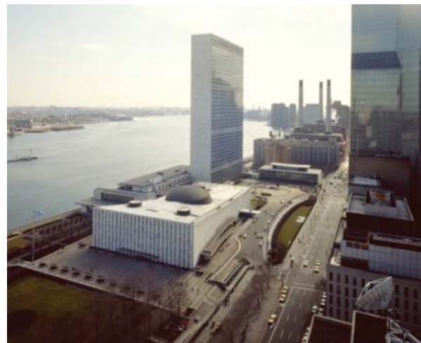
UN Headquarters, North-side view
