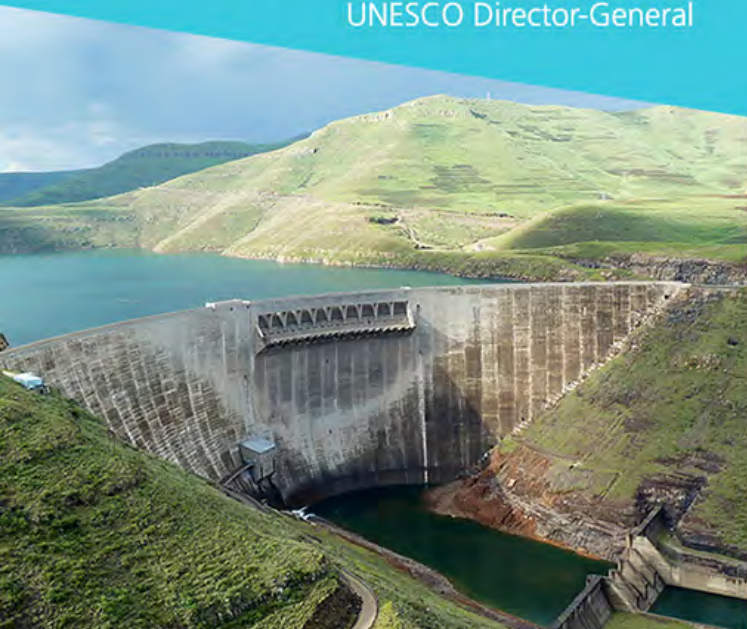
"Creative Commons Africa's highest and second-largest dam (185 m high, 710 m long) by Damien du Toit, www.flickr.com, CC BY-NC-SA 2.0
