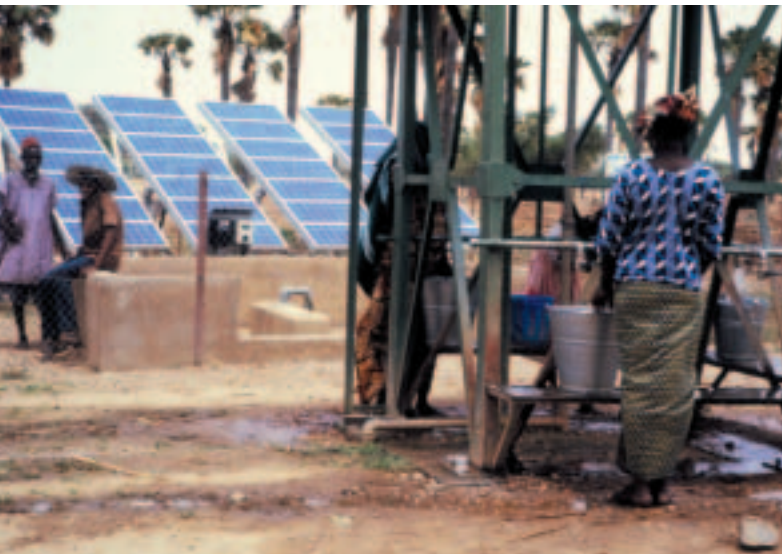
Collecting buckets of water from a solar-powered pumping station. This saves village women and girls from having to walk several kilometres each day to fetch water
